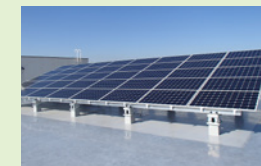
Solar panel installation
